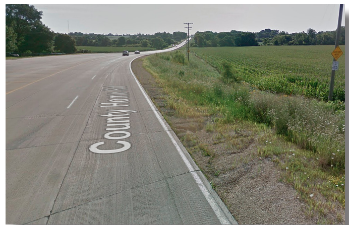
Example of a >800 ADT route that would require the addition of a bike facility to safely accommodate a cyclist. Routes without a shoulder at all should be avoided. Source: maps.google.com , streetview.
