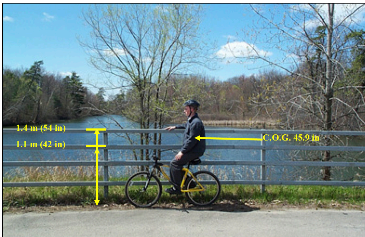
Figure 9: Example of Cyclist Beam Guard to aid on Slopes, not fit to stop a vehicle. Source: NCHRP, Determination of Appropriate Railing Heights for Bicyclists
