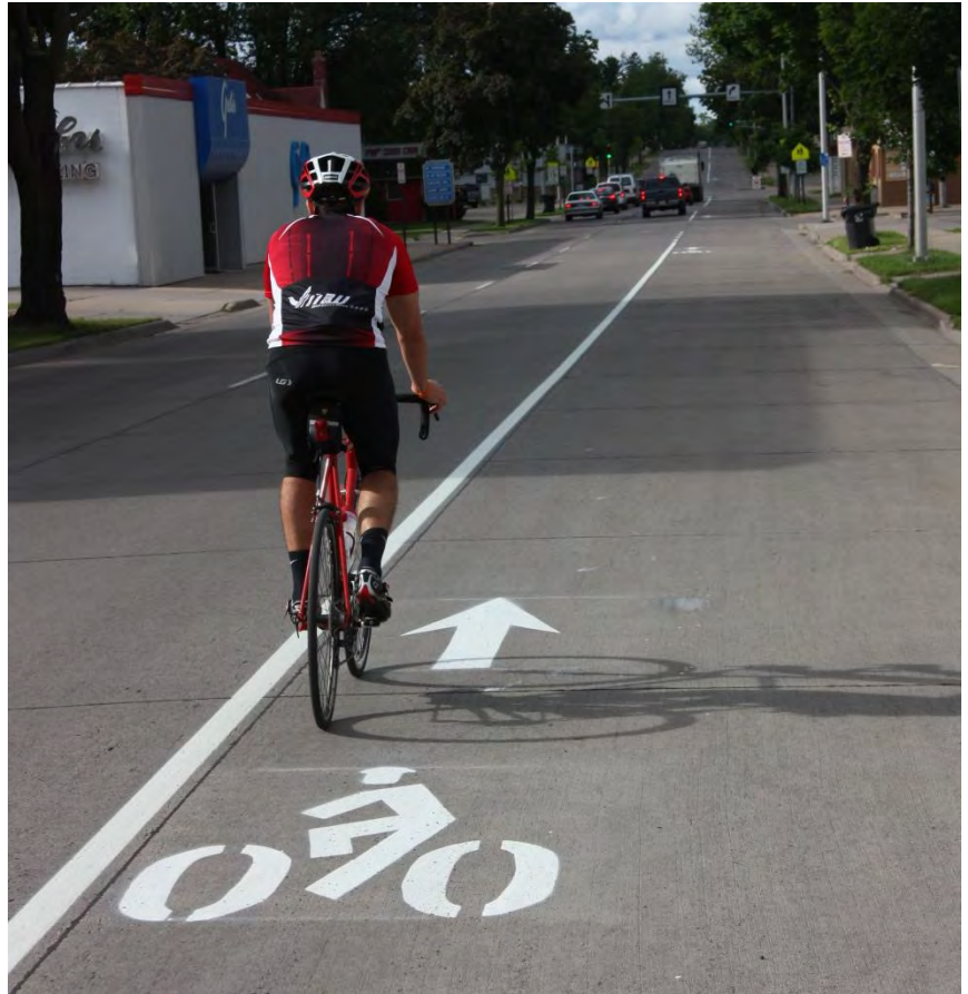
Excess capacity on 3 rd Avenue in Wausau allowed a “road diet” to be performed to convert the right-most travel lane to a wide bike lane. Photo by Pat Peckham, City Pages.
